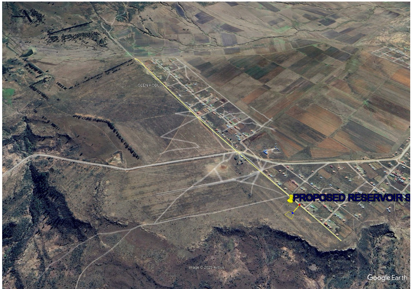
Figure 2D: Leg one reticulation mainline.
